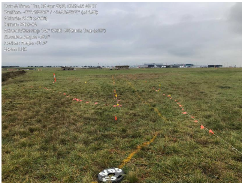
Figure 6: Example of flagging installed prior to works
