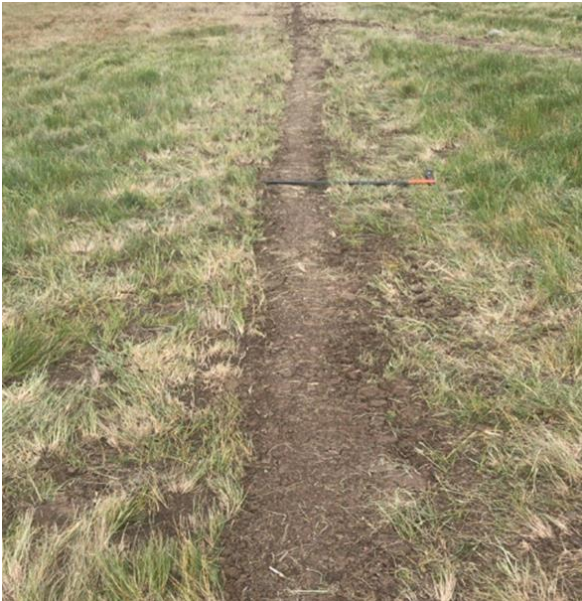
Figure 5: Example of completed trench and temporary impact area
