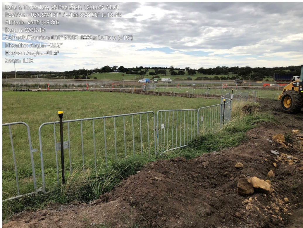
Figure 7 Examples of exclusion fencing and signage
